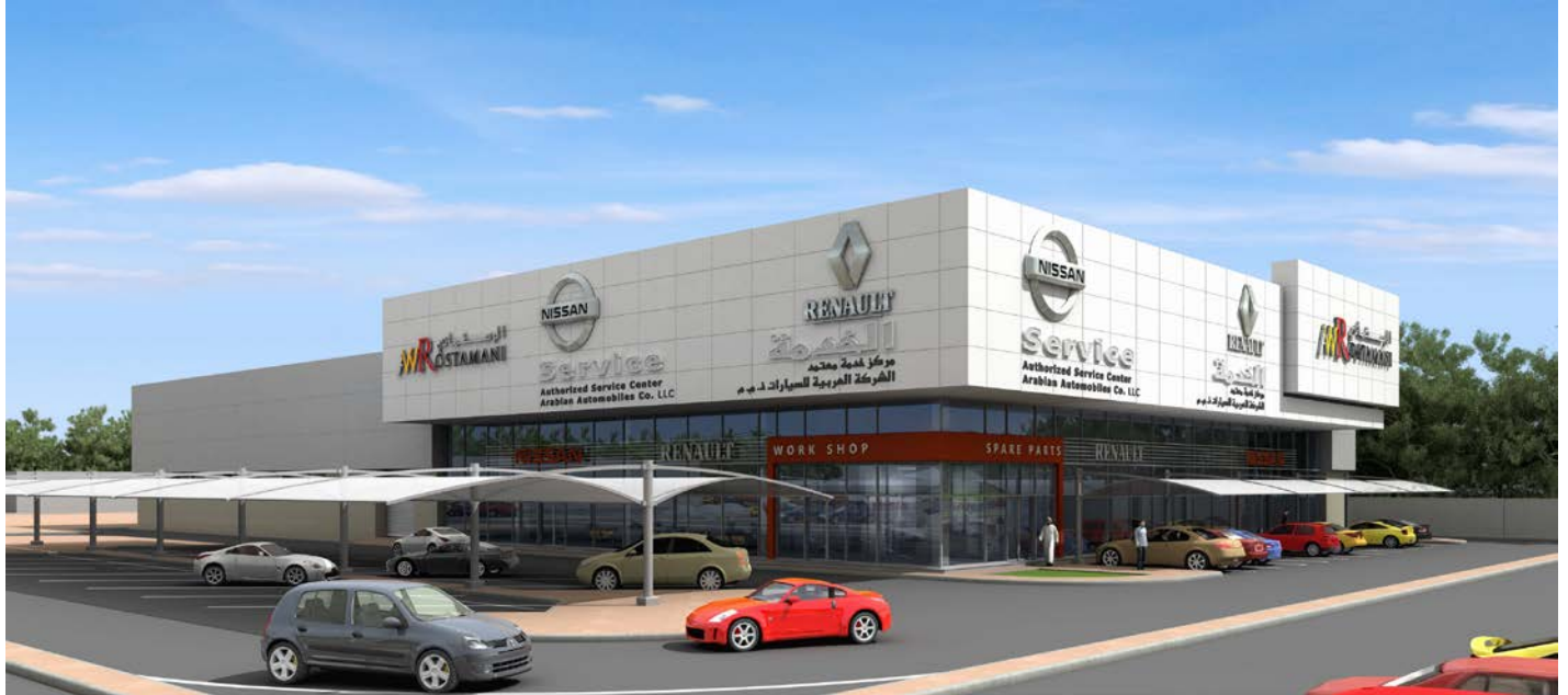
Infinity Showroom & Service Centre on Plot No. 47, Al Rukaa Al Hamra, Sharjah, UAE for M/s. Arabian Automobiles Co. (LLC) – Phase II
