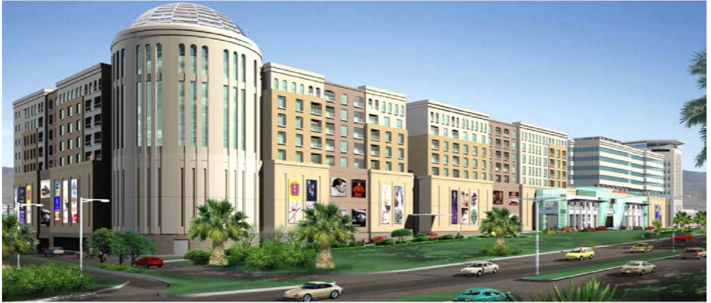
Tilal Complex at Al Khuwair, Muscat, Sultanate of Oman for M/s. IBN Khaldun Al Madina Engineering Consultants
