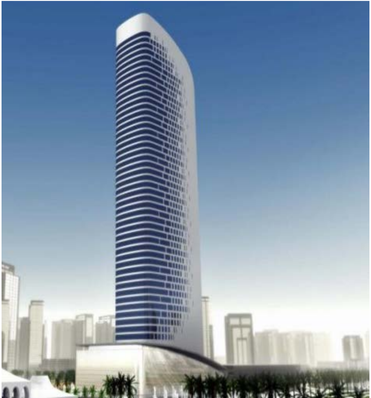
Bay Gate Office Tower on Plot No. BB A01.003 at Business Bay, Dubai
