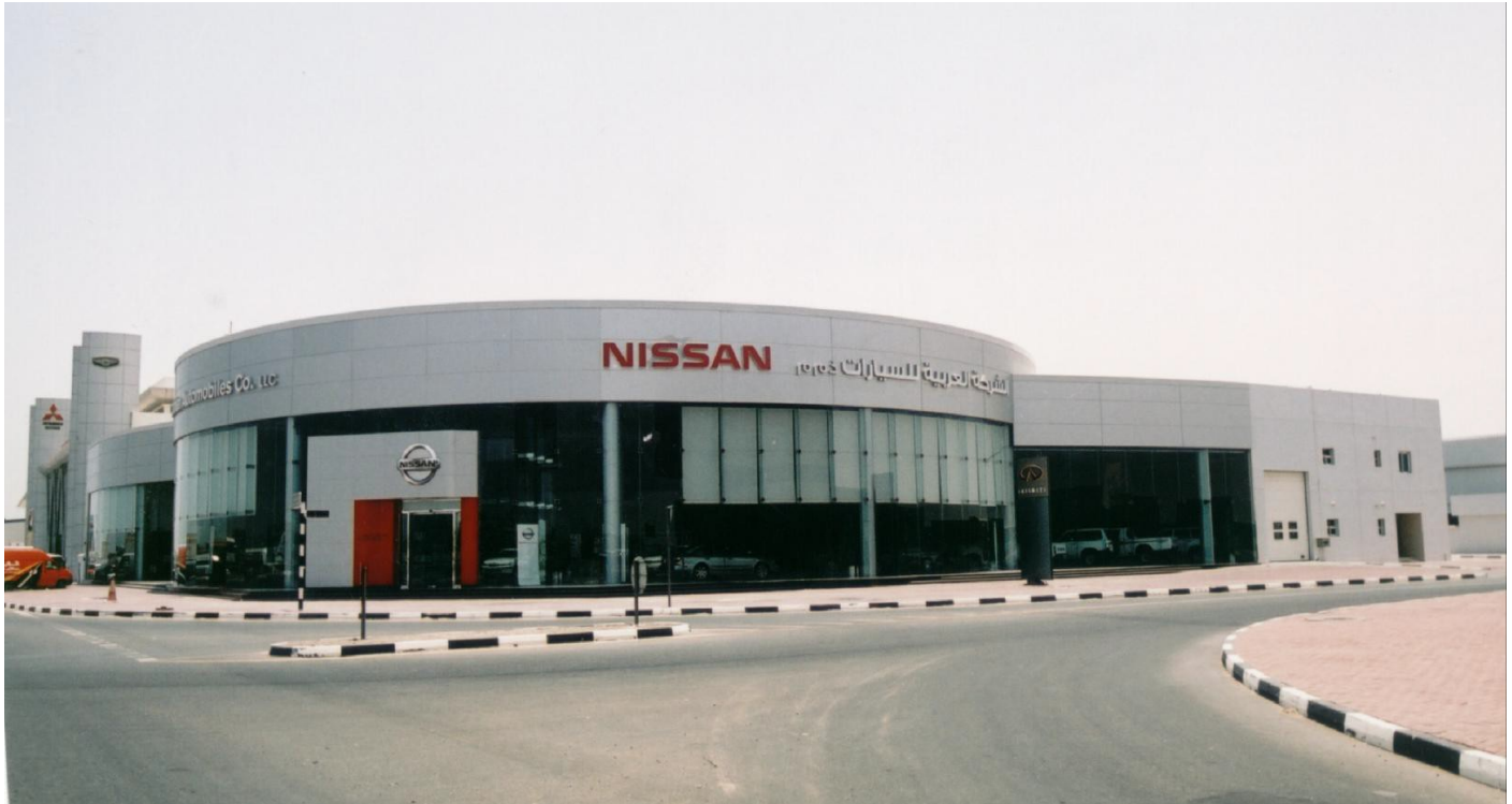
Show Room & Workshop on Plot No. 1560-& 1561 at Al Goze Consultant: Al Hashemi Consultants
