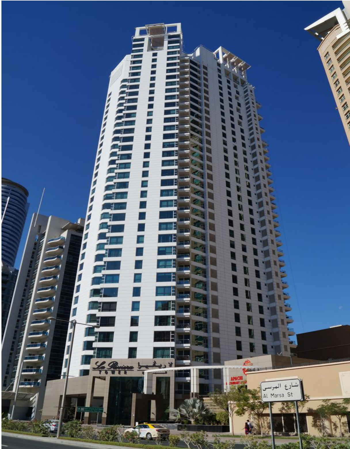
3B+G+36+R) Residential Building – LA Riviera Tower on Plot no. 4U at Dubai Marina for M/s. B&M Fz Co.
