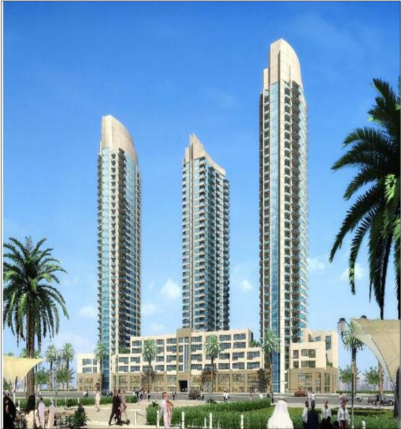
E-34 Burj Development – The Lofts on Plot 18, Burj Dubai for M/s. Emaar Properties PJSC
